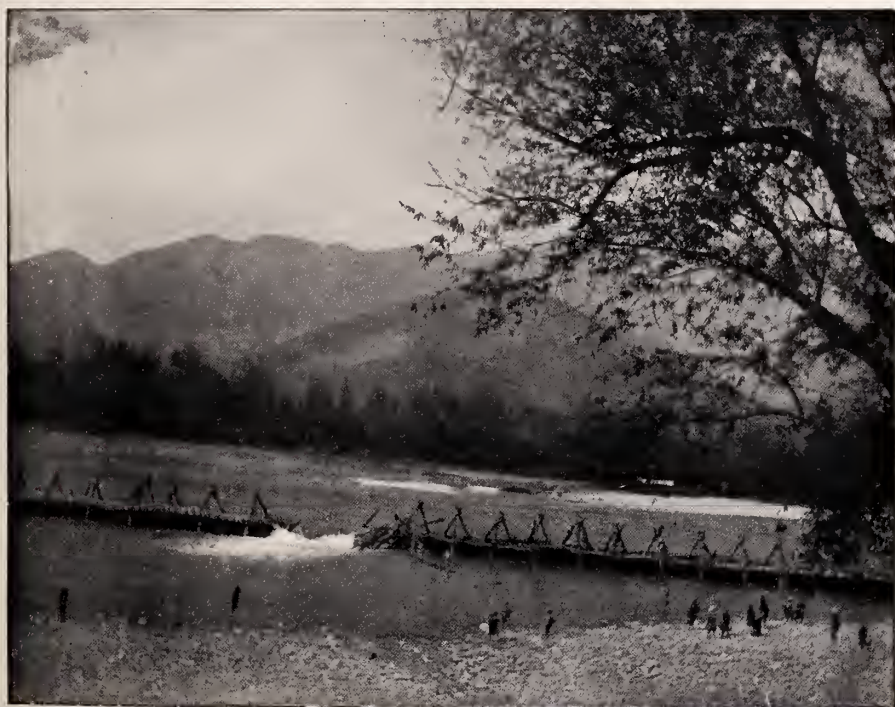
First breach in the 'barrage' at Kwanhien (to be followed by its total removal), whereby the waters of the Min are admitted into the hitherto dry North-eastern irrigation system. This 'barrage' is removed each year in April and replaced again in November.
